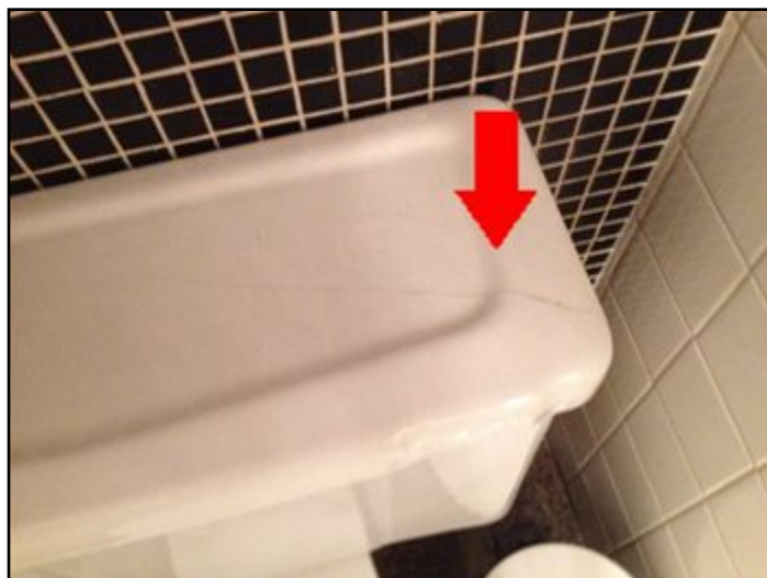
Cracked lid noted
