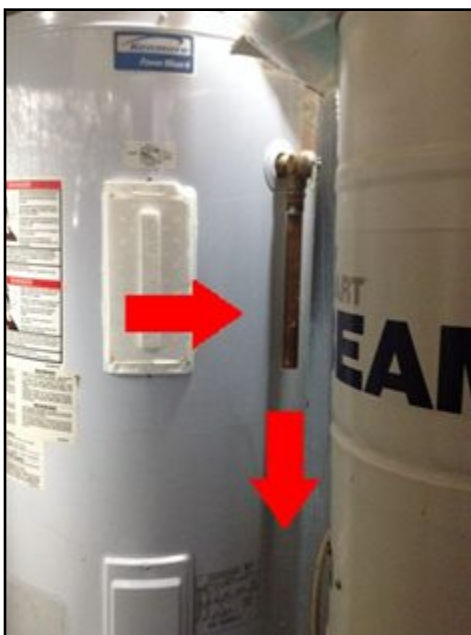
Discharge tube to short
